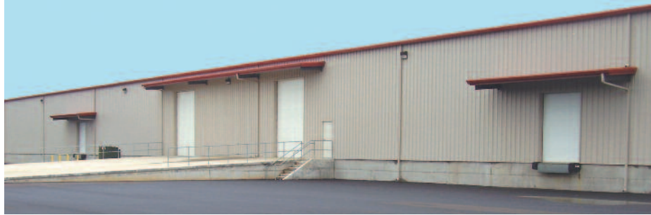
50,000 sq. ft. industrial building
