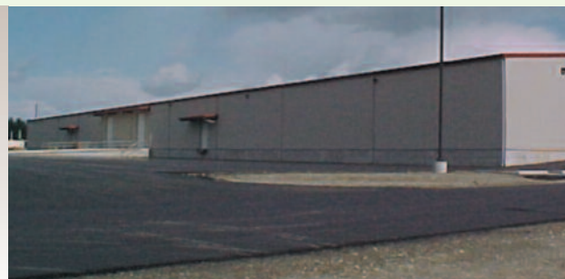
Truck parking and laydown yard
